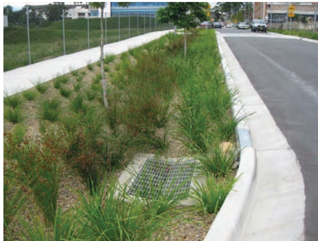
BIO-SWALE WITHIN ROAD VERGE
