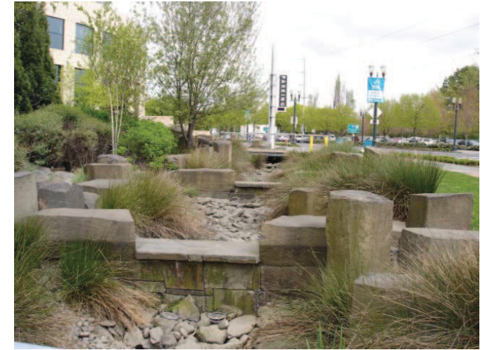
INTERMITTENT CREEK BED DRAINAGE
